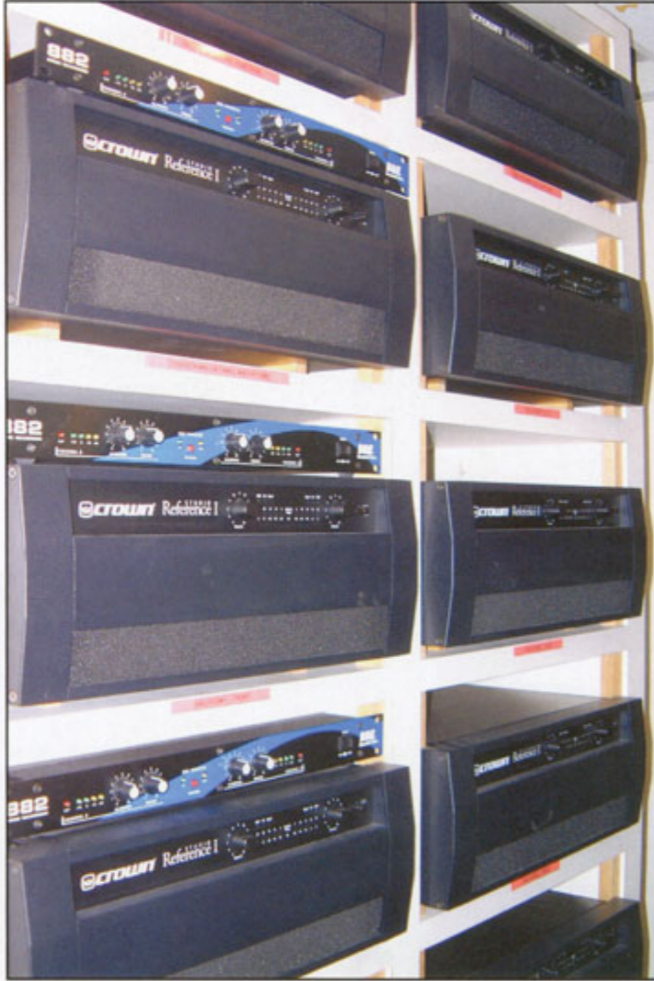
Left: The Banquet Suite control room.
